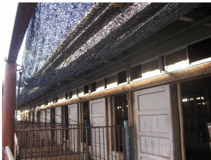
The ceiling set up with cheesecloth
